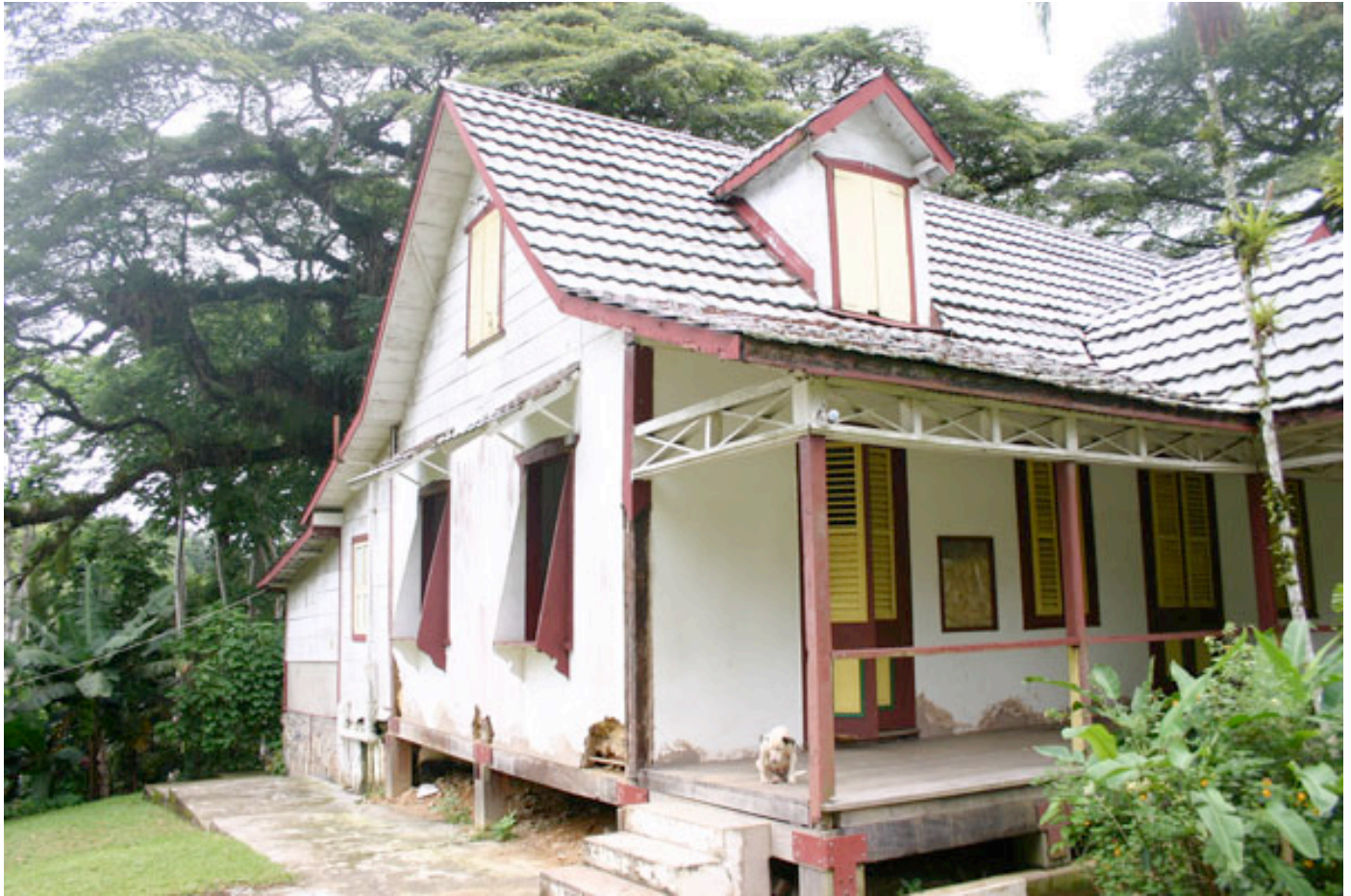
fig. 5. Ajoupa-type elevation of floor, half-hipped roof (i.e., pitched roof with modified angle adjusting steepness), and dormer window. Wattle-and-daub construction visible on side wall, Compte de Lopinot House, Lopinot, Trinidad.
