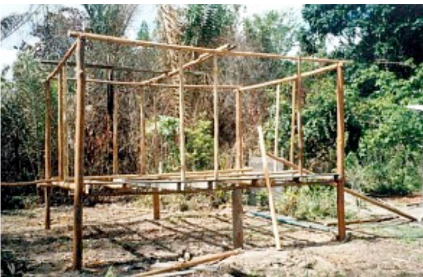
fig. 2. Traditional ajoupa construction with floors elevated on wooden posts, Pakuri Arawak Territory, Guyana. Photographs by Damon G. Corrie.
