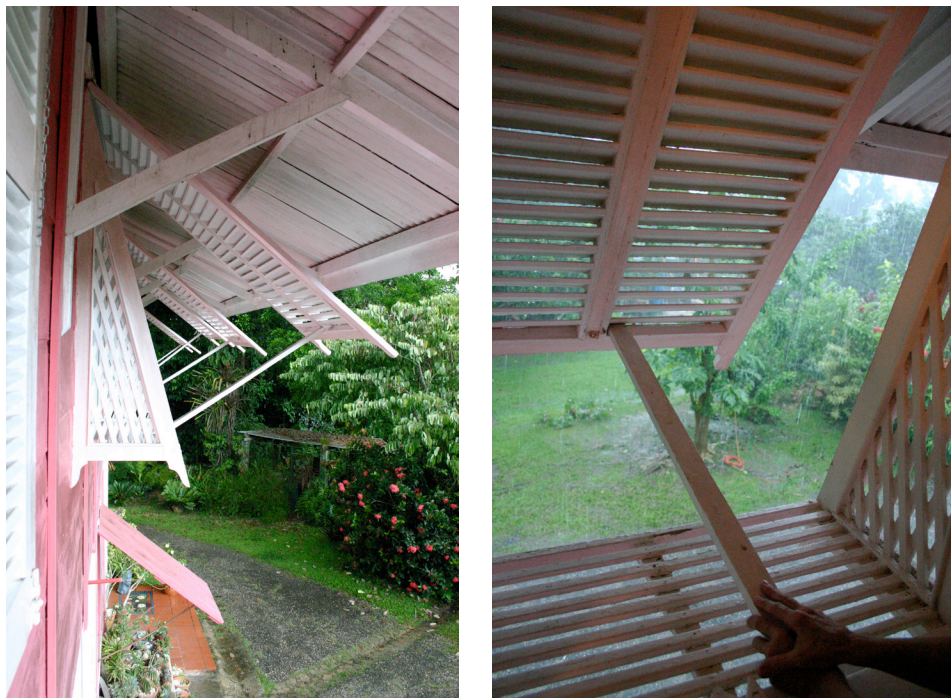
fig. 4. Demerara windows aerated through jalousies, side lattices, and underside slats of tilted window box, "Ajoupa" (home of Rory and Bunty O'Connor), Freeport, Trinidad. Photograph by author.
