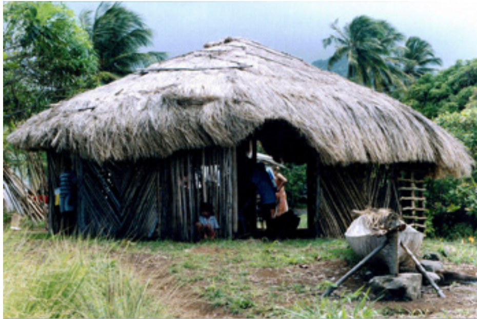
fig. 1. Traditional Carib structure, used as a meetinghouse, with vertical and diagonal picket walls, Carib Territory, Dominica. Photograph by author.
