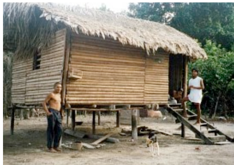
fig. 2. Traditional ajoupa construction with floors elevated on wooden posts, Pakuri Arawak Territory, Guyana. Photographs by Damon G. Corrie.
