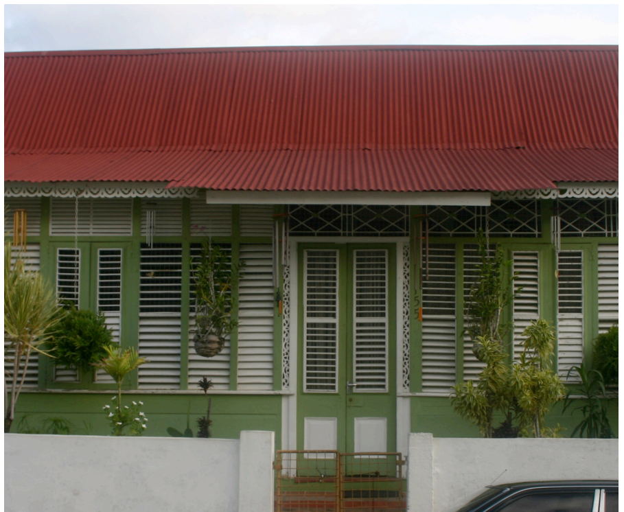
fig. 3. Elevated house with jalousie window walls, and French doors, Port-of-Spain, Trinidad. Photograph by author.
