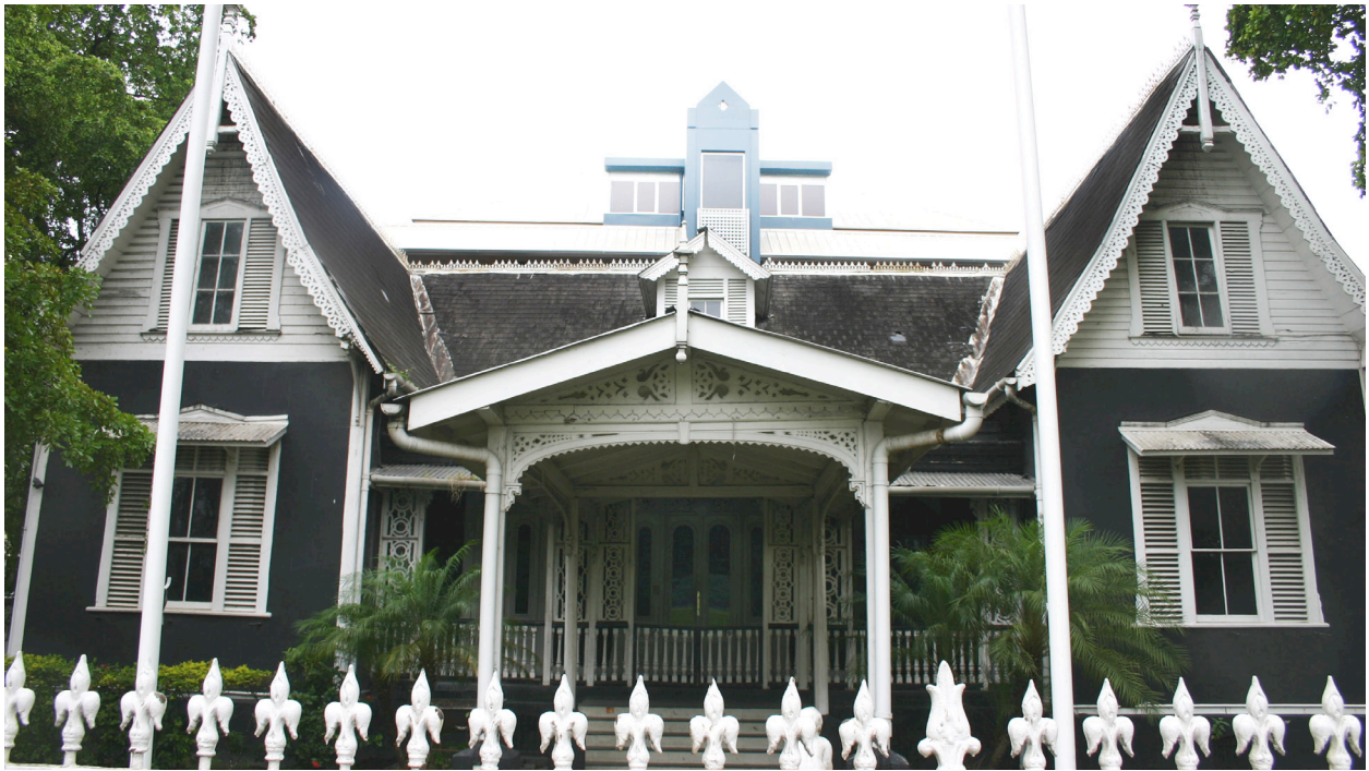
fig. 9. Openwork pedimented porte cochère, front porch and bargeboards above bay windows, George Brown House, Queens Park Savannah, Port-of-Spain, Trinidad. Photograph by author.
