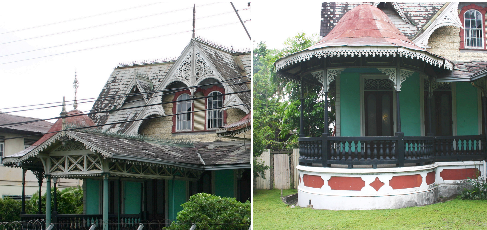
fig. 13. (Left) Openwork bargeboards, pinnacles/finials and wrought iron ridge crests on main roof and pedimented porte cochère; (right) gingerbread Chinese pavilion, on hollow plinth, extending porch, and openwork transoms (jalis) over French doors, Boissiere House, Queens Park West, Port-of-Spain, Trinidad. Photograph by author.
