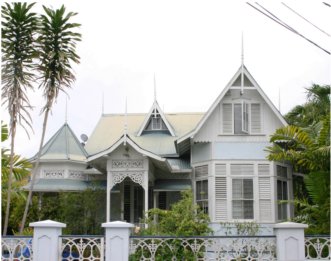
fig. 8. Jalis on portico (center left) and along tops of porch and Chinese pavilion (left); other fretwork webs lintel of portico (center left); pinnacles (i.e., finials) at ridge ends, Gingerbread House bed and breakfast, Port-of-Spain, Trinidad. Photograph by author.
